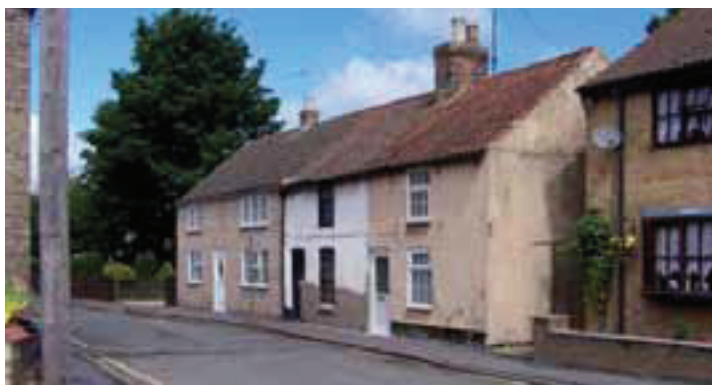
Replacement of windows and doors with uPVC, Caroline Street
