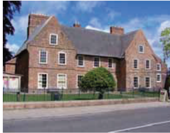
Alford Manor House, West Street
