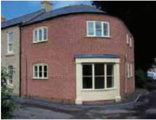
New development, Corner House on Ranters Row
