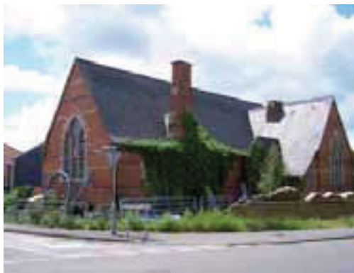
Derelict school building fronting West Street
