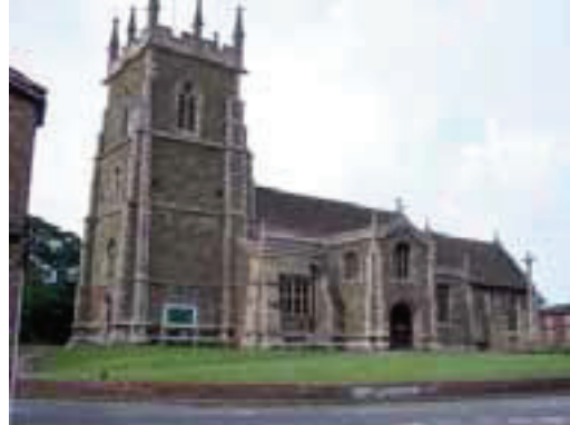
St Wilfred's Church, Church Street
