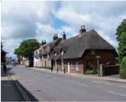
Nos. 116-118 West Street – view south west
