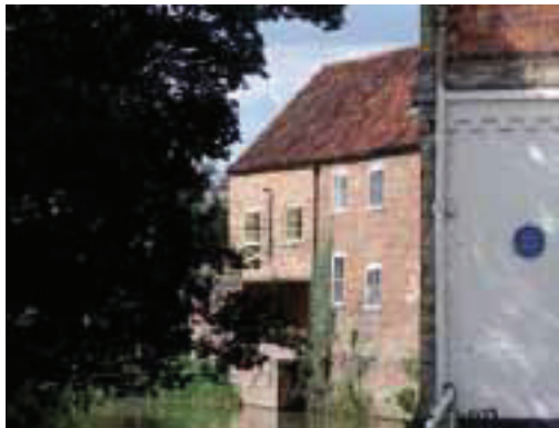
Rear of No.25 Bridge Street
