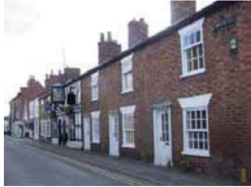
Nos. 55-71 North Street
