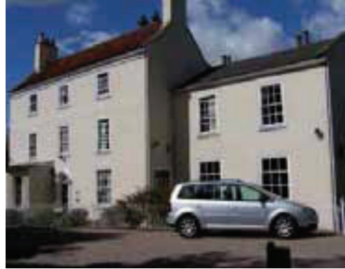
Banovallum House, Manor House Street
