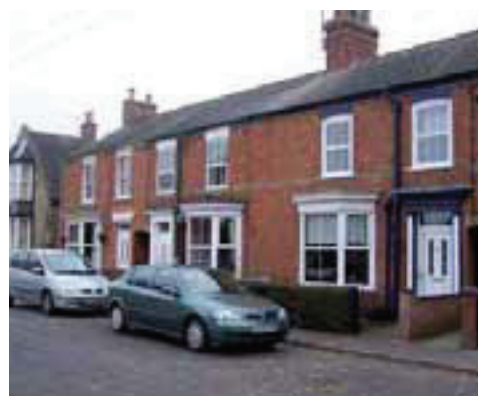
Nos. 7-13 Croft Street
