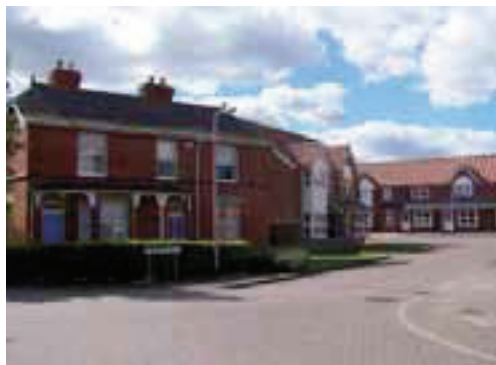
Jubilee Way – former station house in foreground
