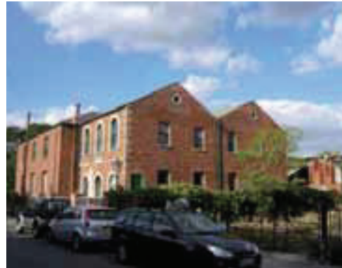
Congregational Chapel, Queen Street
