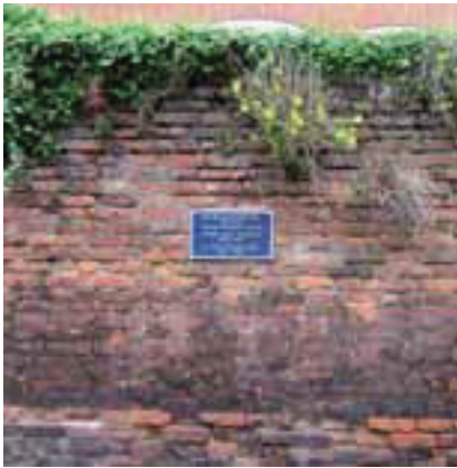
Old brick wall, School House Lane
