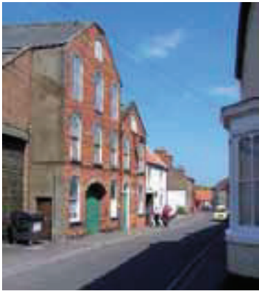
Nos. 57-67 Queen Street
