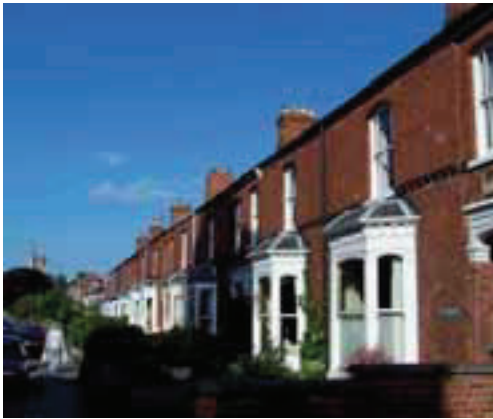
Eastgate – view east
