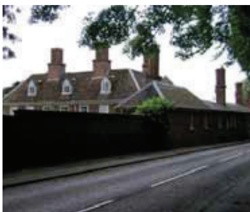
Thorpe Hall, Elkington Road
