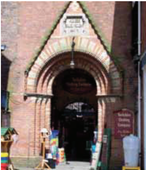
Market Hall door detail
