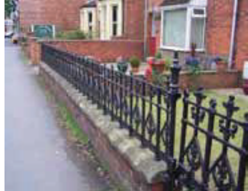
Railings at Nos. 15-23 (odds) Witham Road
