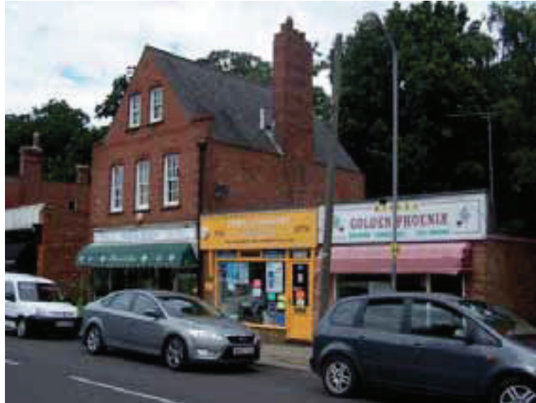
Station Road – poor quality shopfronts
