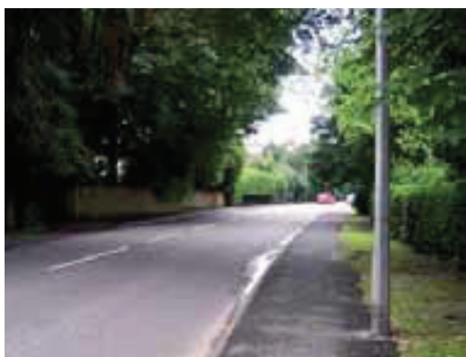
East Street – view north east
