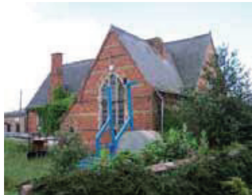
Derelict former Boys School, West Street
