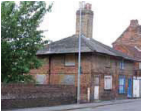
Derelict Listed Buildings, Nos. 12 & 14 South Street
