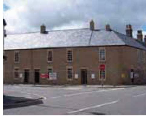
New development, corner of West Street and Hamilton Road
