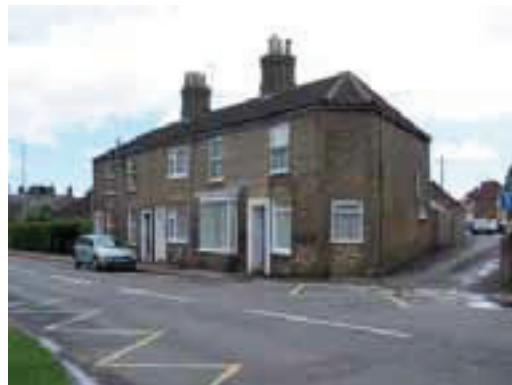
Nos. 61, 63, 65 and 65a South Street
