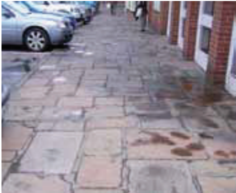
York stone paving, South Market Place
