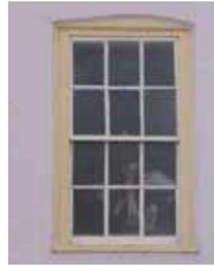
Window detail at Nos. 15/17 Bridge Street
