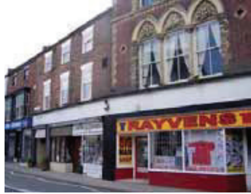
Poor quality shopfronts along Bridge Street
