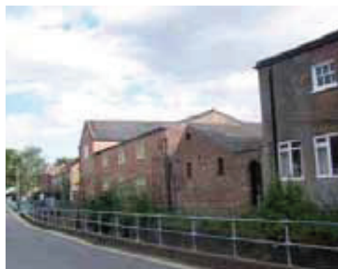
Banks Road – view east
