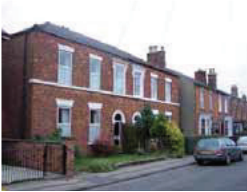
Contrast between traditional windows and poor modern replacements
