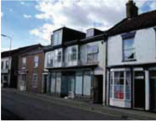
Vacant premises along East Street
