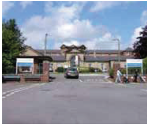
County Hospital, High Holme Road
