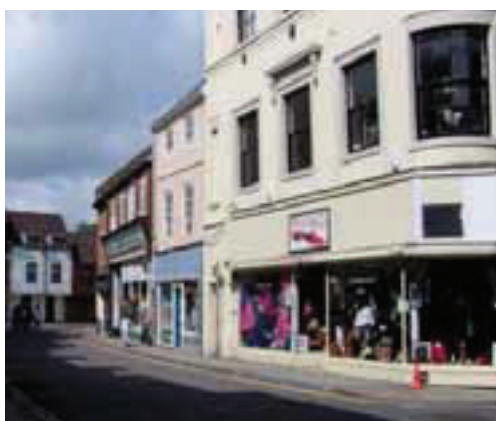
Poor quality shopfronts
