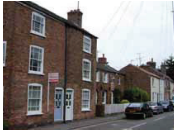
Nos. 5-21 Edward Street
