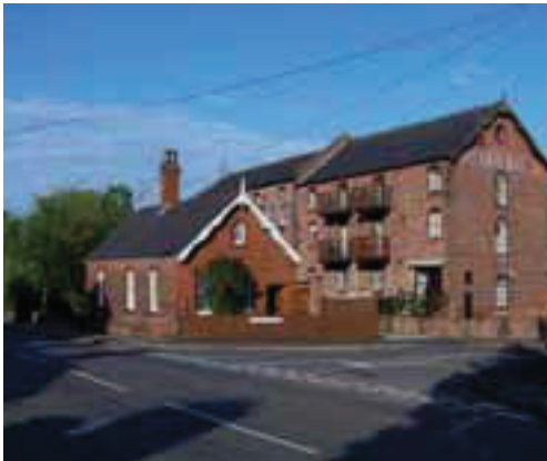
Crown Mills, Ramsgate Road
