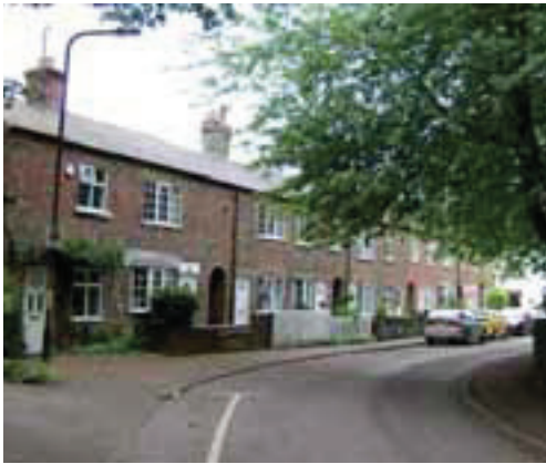
Nos. 73-91 Crowtree Lane
