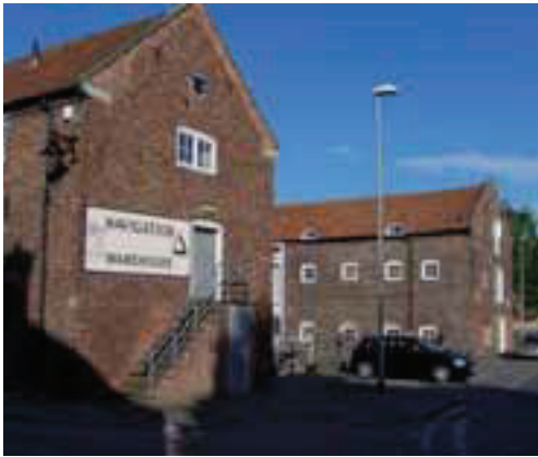
Navigation Warehouses, River Head Road
