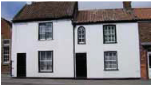
Stucco used at Nos. 8-10 Church Street
