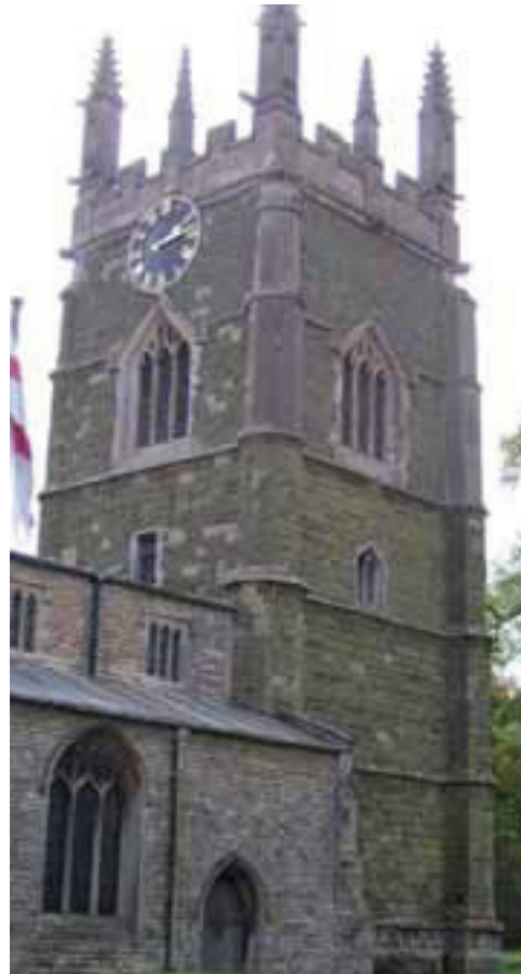
Green stone or Spilsby sandstone in use on St. James's Church Tower
