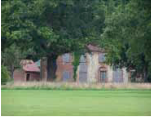
Outbuildings to the Old Manor House, Spa Road
