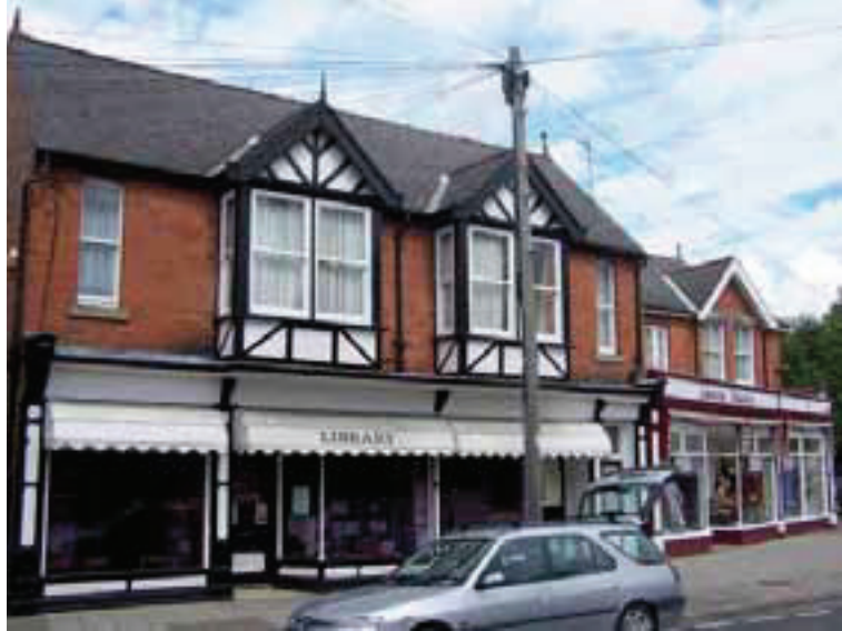
Nos. 1 & 2 Station Road – good traditional shopfronts which frame the shop windows and support the upper floors
