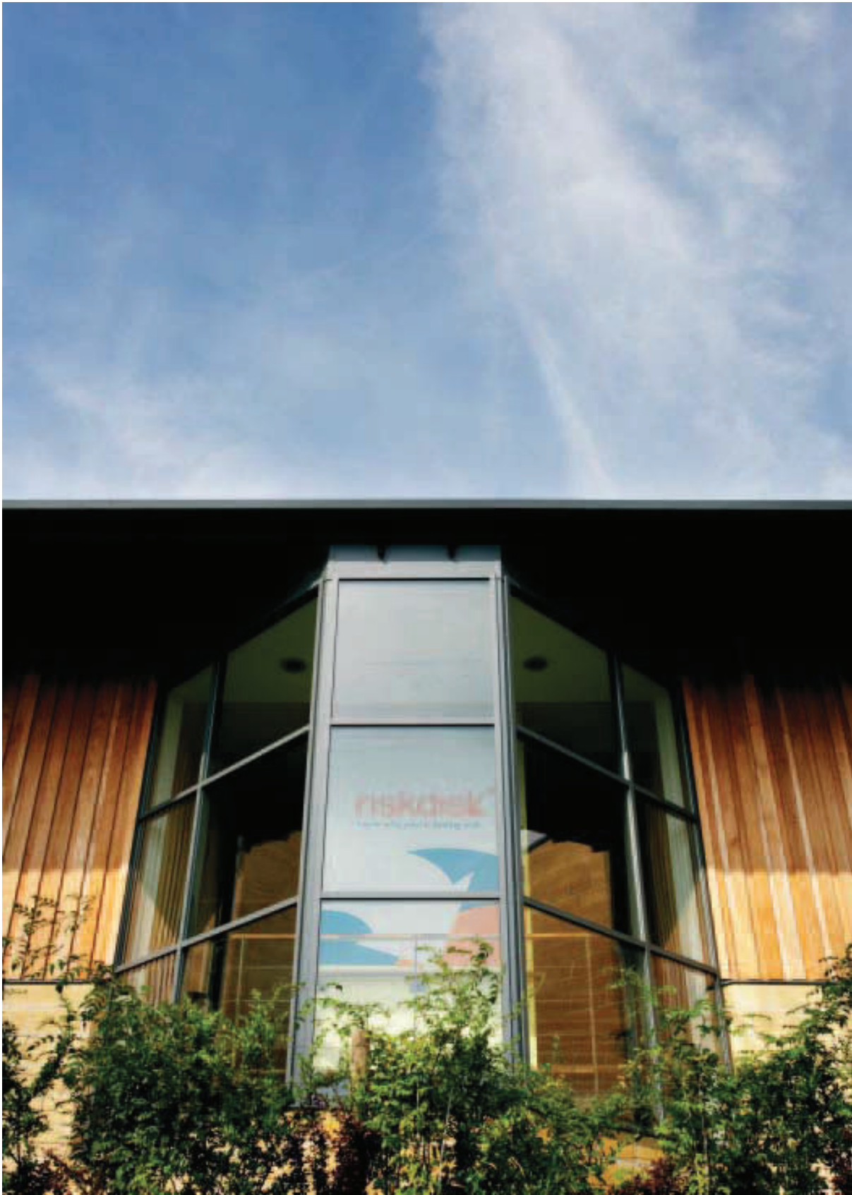
PICTURED: SHERWOOD ENERGY VILLAGE, OLLERTON, NOTTINGHAMSHIRE.
