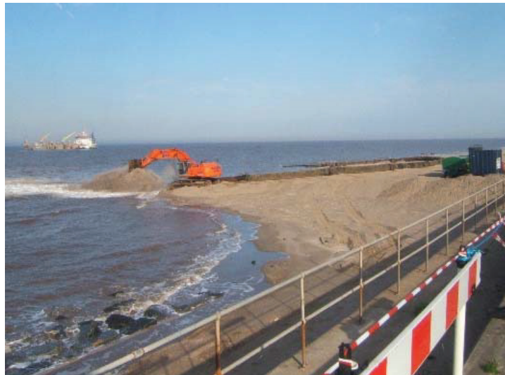
Photo 3 – Onshore Pumping of Beach Nourishment
