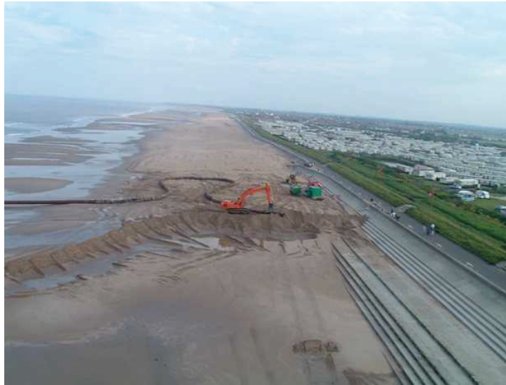
Photo 1 – Aerial view of the beach at Lincshire during nourishment
