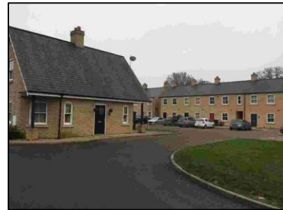
Fig. 6: Back of The Anchor
