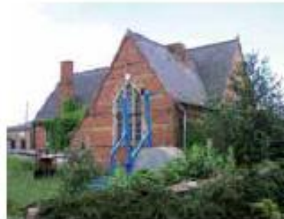
Derelict former Boys School, West Street
