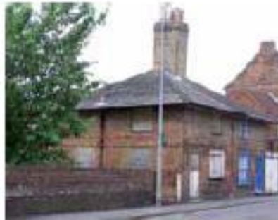
Derelict Listed Buildings, Nos. 12 & 14 South Street
