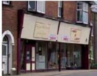
Poor quality shop fronts along West Street
